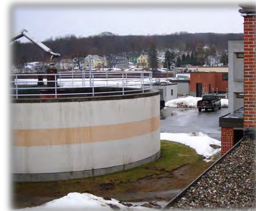
Primary Digester - Rutland, VT 1.2M Gal. Digestion Volume
